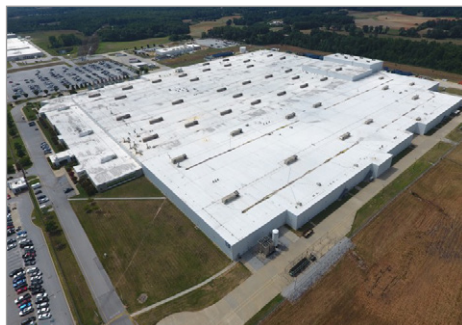
ZF plant in Gray Court, South Carolina
